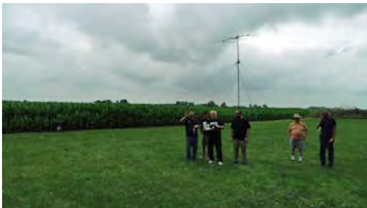
Erecting the 6 meter Yagi
