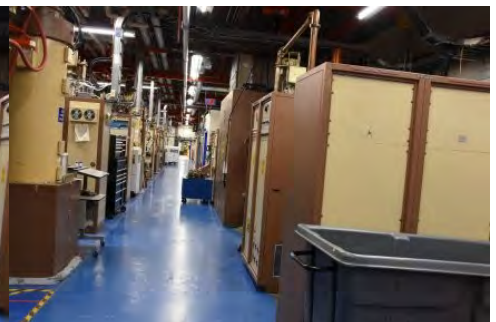
Row after row and isle after isle of control circuits, power supplies, amplifiers & klystrons supply the millions of Watts and up to a trillion Volts to the giant particle accelerator
