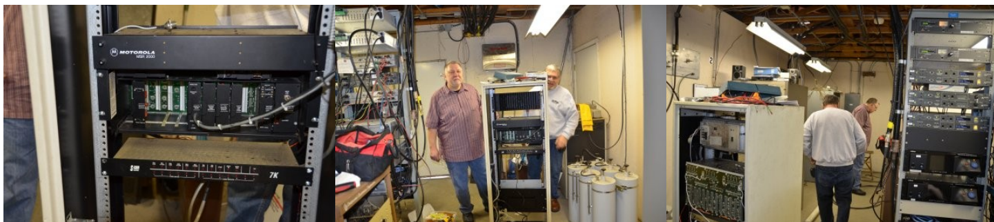
A view of the Motorola MSR2000 repeater and SCom controller... the 100% duty cycle power supply and 100 Watt final amplifier are not visible.
