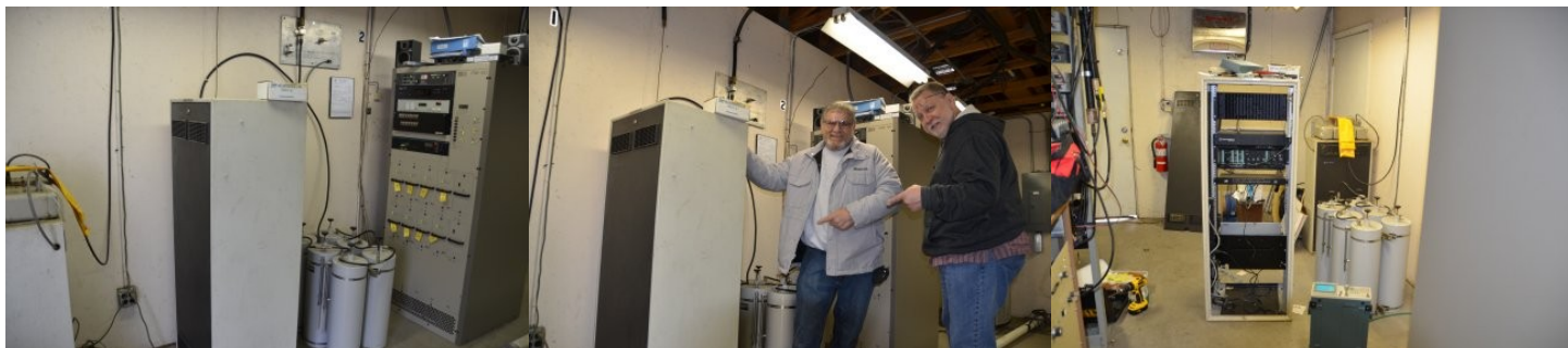
The 145.130 repeater and duplexers sitting in front of the WKCC broadcast transmitter
