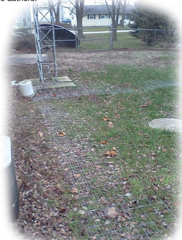
Inverted - L Ground screen (Fig 1) made from 28 inch fencing Layed on ground.
