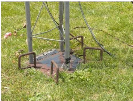
Close-up detail of the custom made tower base plate
