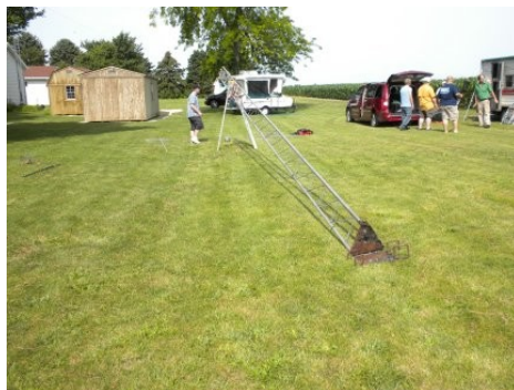
Prepping the VHF/UHF tower
