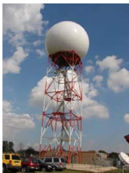
The state-of-the-art Doppler weather radar antenna
