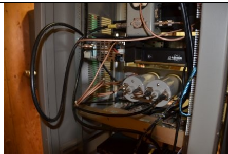
Rear view of the new 444.800 repeater during installation
