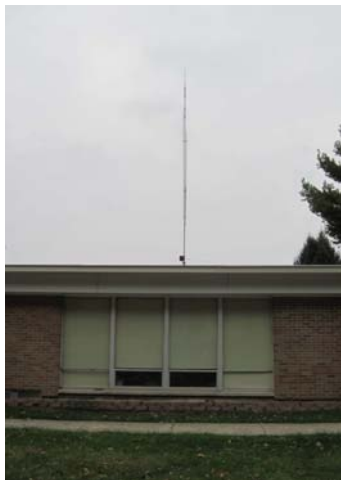
New Antenna installation at W9GRS
