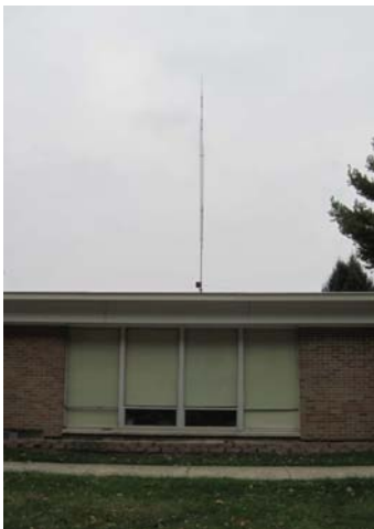
New Antenna installation at W9GRS
