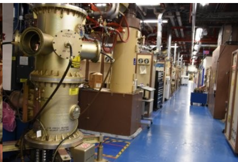
Row after row and isle after isle of control circuits, power supplies, amplifiers & klystrons supply the millions of Watts and up to a trillion Volts to the giant particle accelerator
