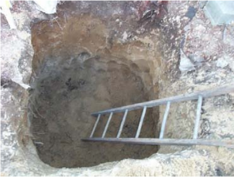
A large free standing tilt over tower requires a LOT of concrete in a BIG hole! -N9RJM
