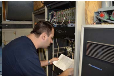
Bill N9OE interfacing the Echolink equipment to the KARS .34/.94 repeater
