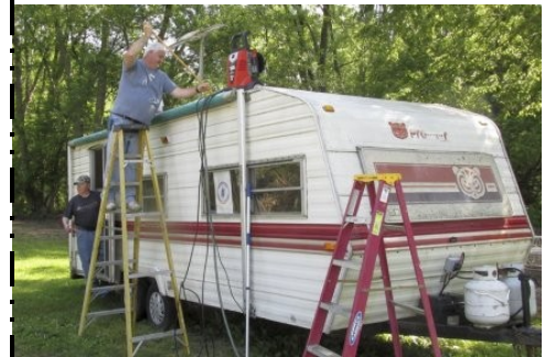
Kevin KC9QXV applying fresh roof sealer
