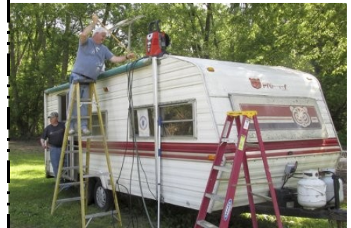
Kevin KC9QXV applying fresh roof sealer
