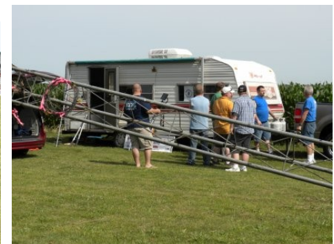
Antenna crew confers prior to hefting the tower in place
