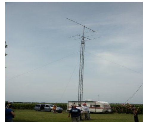
Tower and antennas alongside KARS EmComm unit
