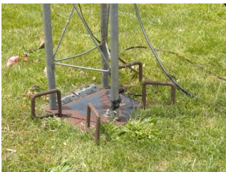
Close-up detail of the custom made tower base plate
