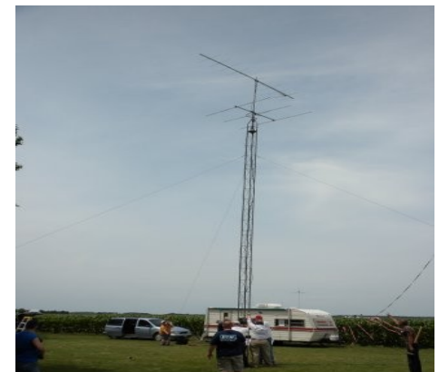
Tower and antennas alongside KARS EmComm unit
