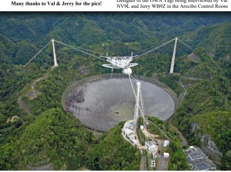
The incredible Radio/Radar Astronomy in Arecibo, Puerto Rico The dish is slightly over 1,000 feet across. The antenna feed, weighing over 900 tons is suspended by cables nearly 500 feet in the air. It was from this antenna feed assembly that Jerry and Val took photos and videos.
