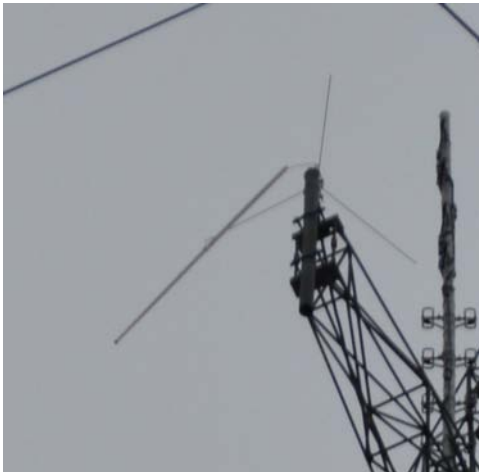
Tornado damaged remote repeater receiver antenna on the Diamond tower Story on page 3
