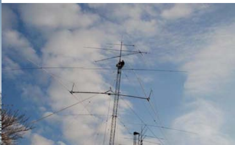
The forty meter Moxon beam on the way up... dwarfs the tribander!
