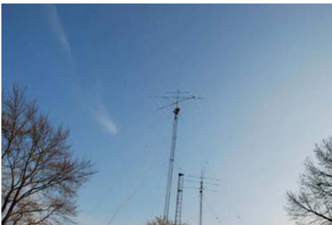
The same antenna at 100 feet Looks pretty small up there!
